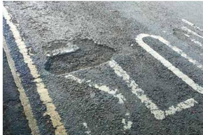
*Figure 21. The poor state of surfaces was a recurrent theme (Photo: Ben Spencer)*
