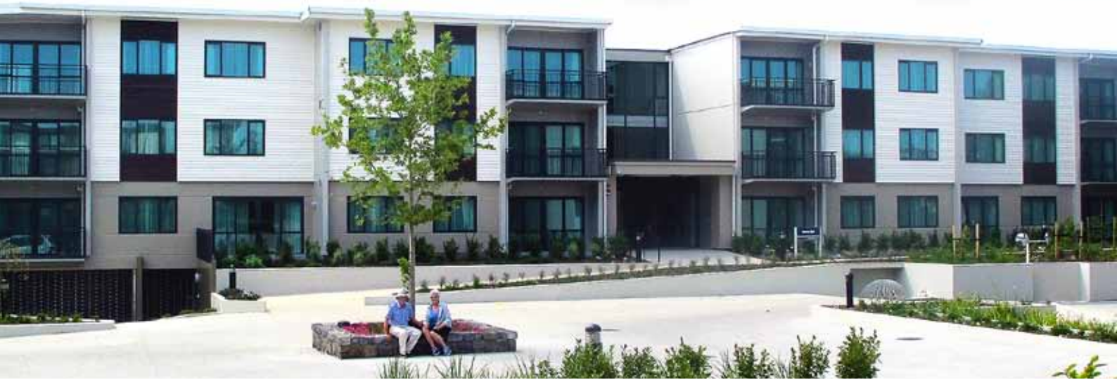
The Newman-Reid Apartments, Selwyn Village
